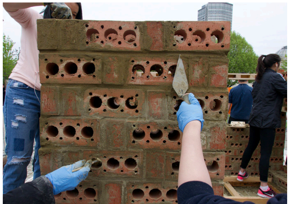
Figure 8: Brick Tea Room, work in progress (Credit: BA ISD students)
